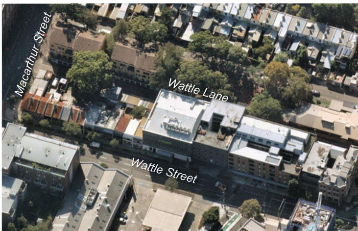
Figure 216 – oblique aerial of 458-468 Wattle Street
