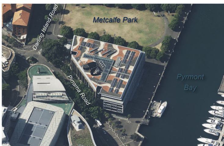
Figure 128 – oblique aerial of 48 Pirrama Road
