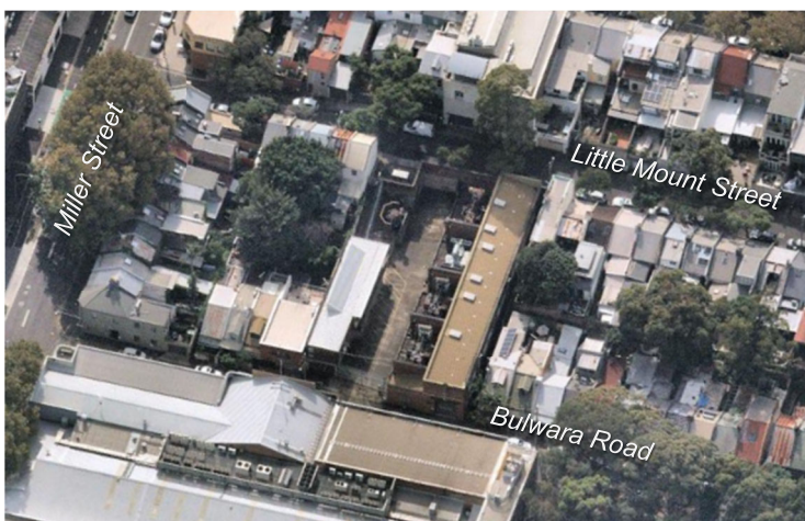
Figure 18 – oblique aerial of 20-28 Bulwara Road
