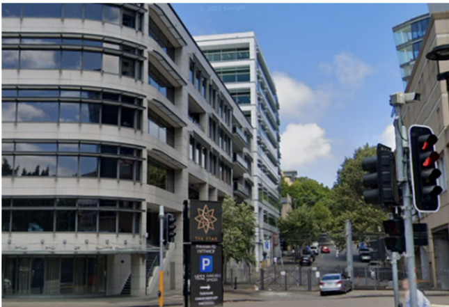
Existing – from Pirrama Road
