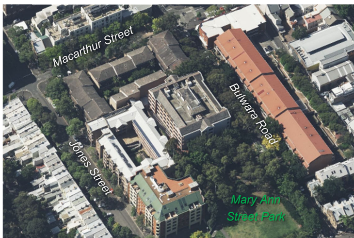
Figure 202 – oblique aerial of 383-389 Bulwara Road
